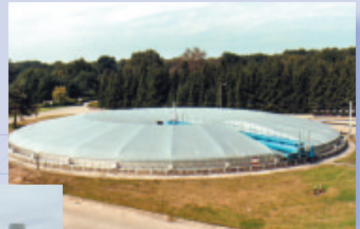
STP Eerbeek, The Netherlands
