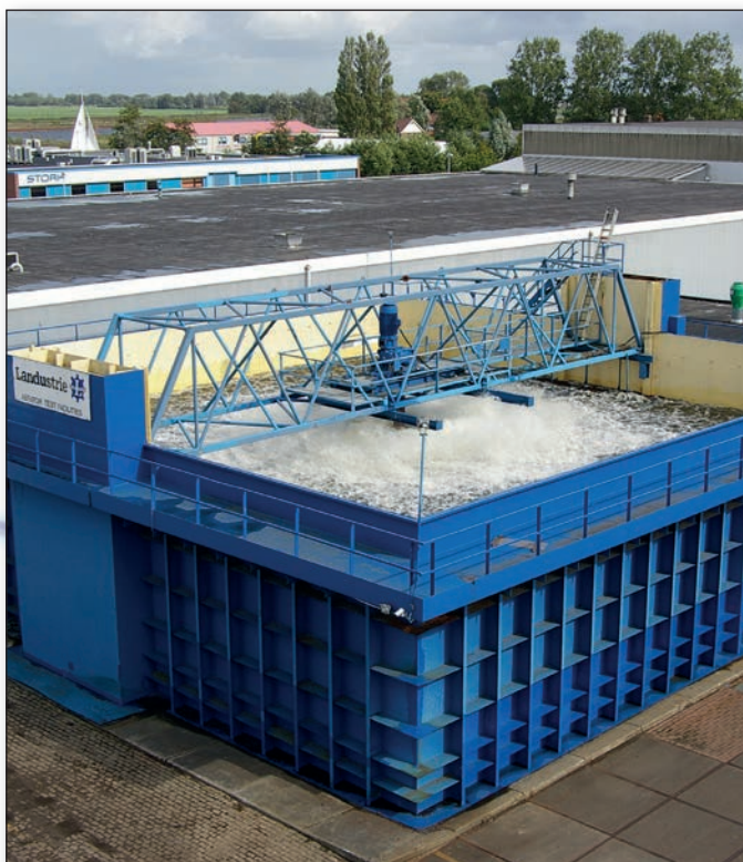
Full-scale aeration test basin at Sneek, the Netherlands
